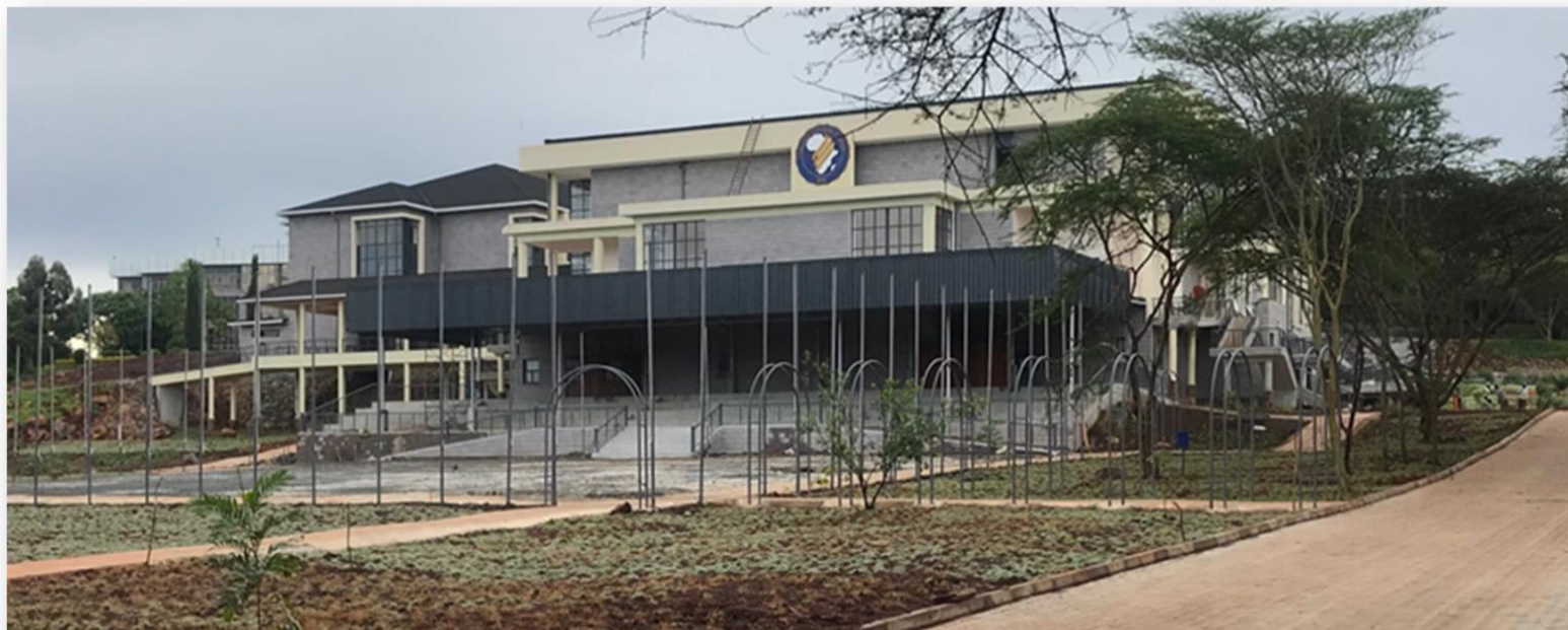
Rear View of the Multipurpose Complex
